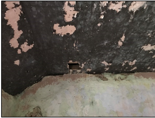
Plate 4-3 Interior of house showing access to the attic
