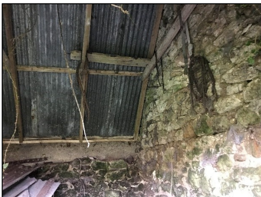
Plate 4-5 Interior of stone shed showing galvanised roof, timber framing, stonework and influx of light.
